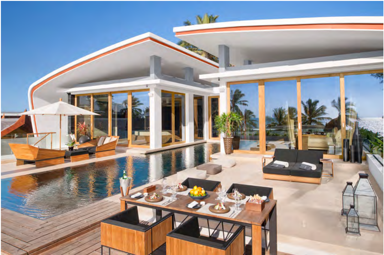
the 'iniala penthouse' is formed by two curving roof structures
